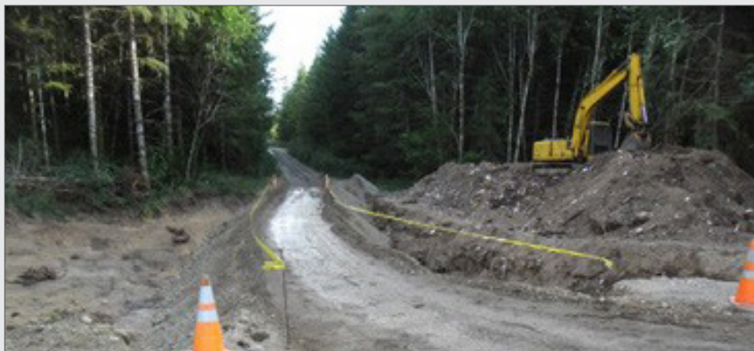
Temporary roadway providing continued access for local residents during construction activities.
