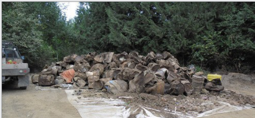
On-site segregation of regulated wastes, allowing for significant transport and disposal cost savings.
