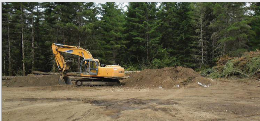
Backfilled area being prepared for surface contouring and reseeding.
